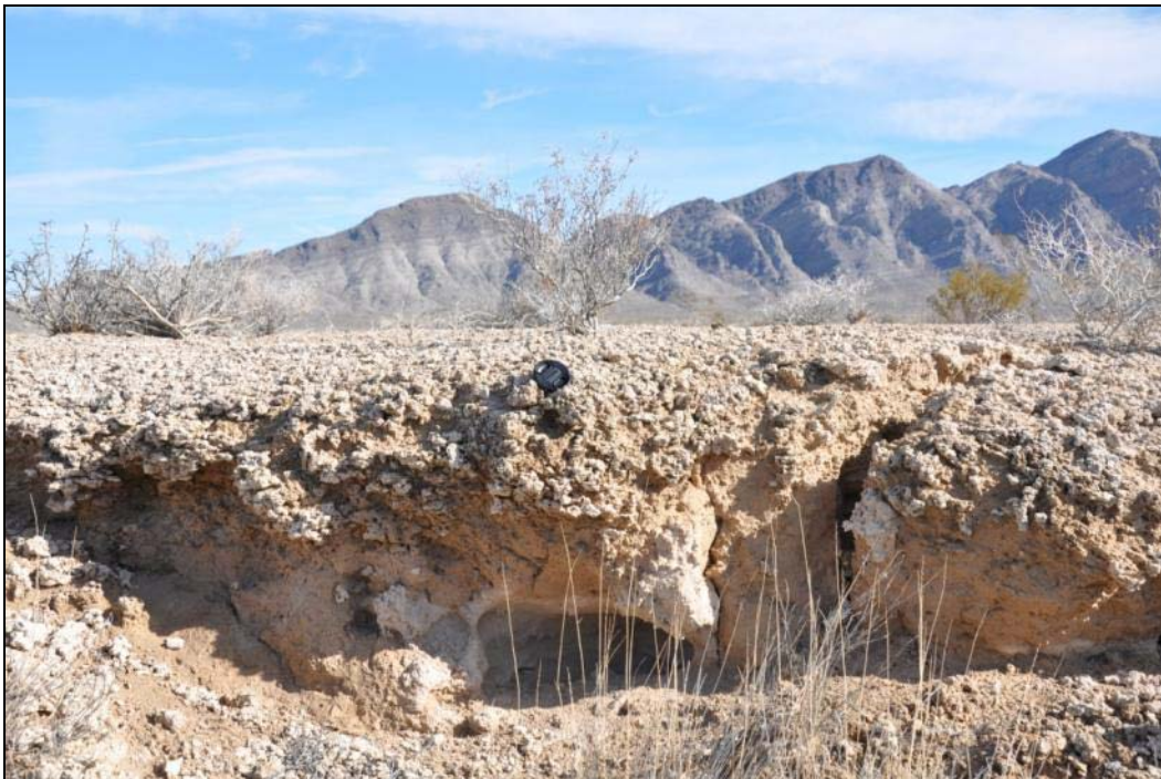
Figure 2-12: A small, ~40cm gully cut bank in Qlv-summit, showing highly-indurated polygenetic soils and a pavement composed of calcium-carbonate rhizolith fragments. This is buckwheat habitat.
